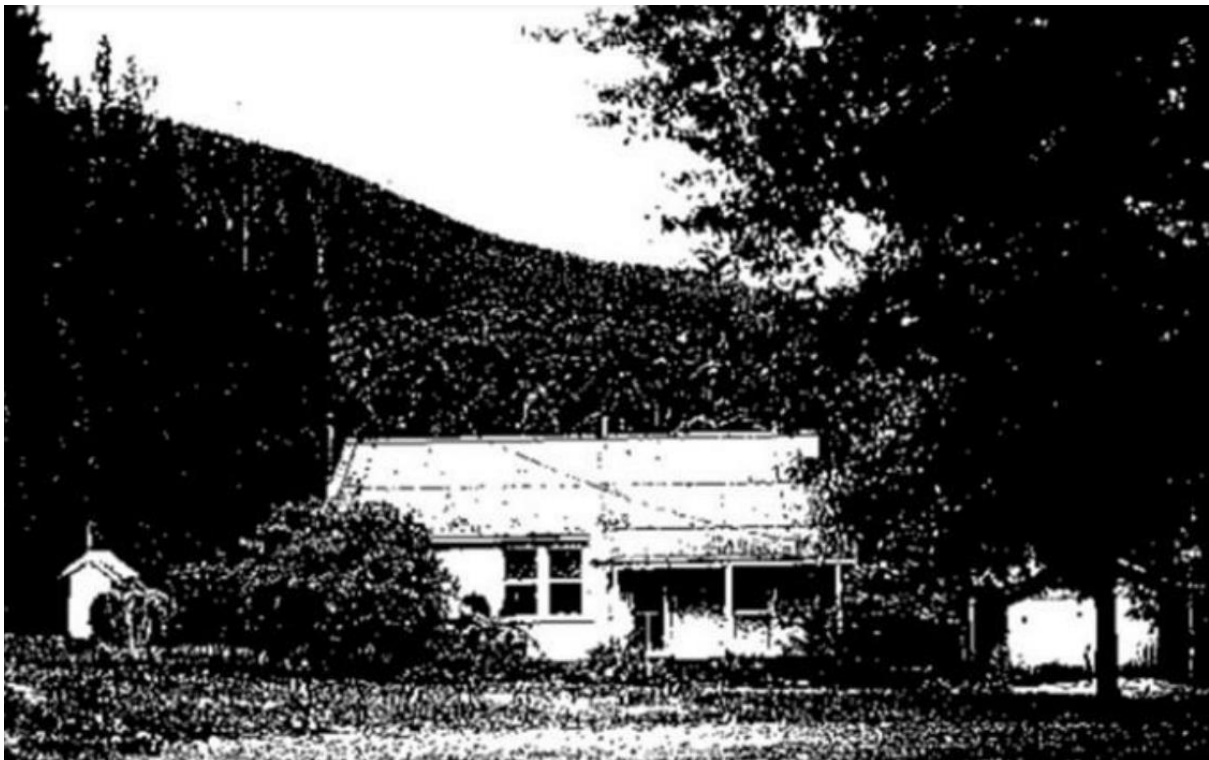
Figure 2 - Former homestead turned caretaker's cottage located south-west of the study area (now demolished) - Image date unknown
